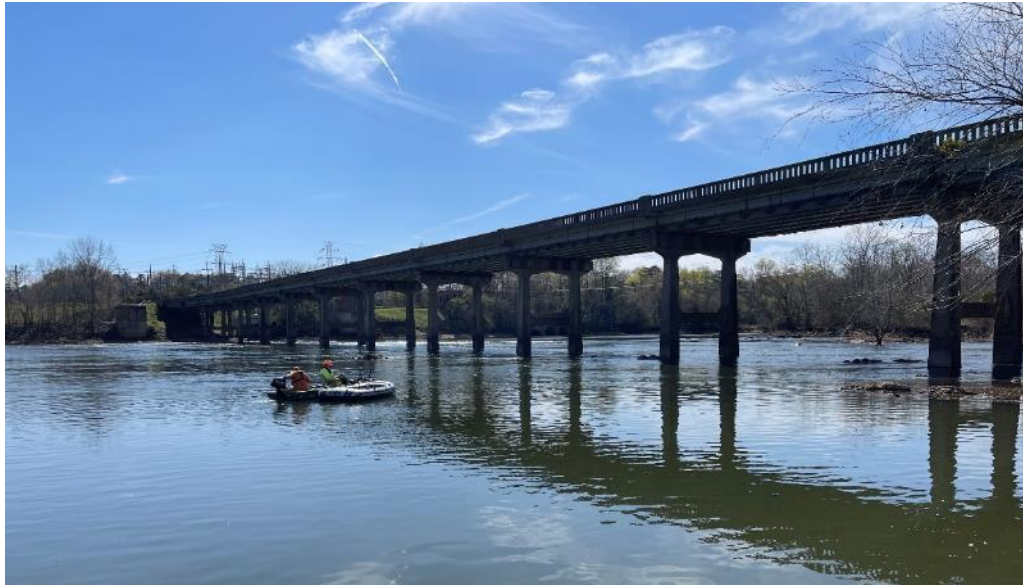
Highway 48 Bridge over Roanoke River
